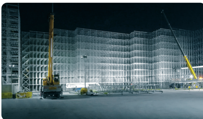
Building of a high-density automated warehouse
